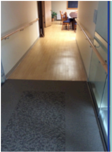
Flooring at the intersection of the two buildings.
